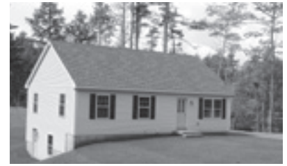
New Construction Gorham — Close to "The Lakes Region" $218,900
