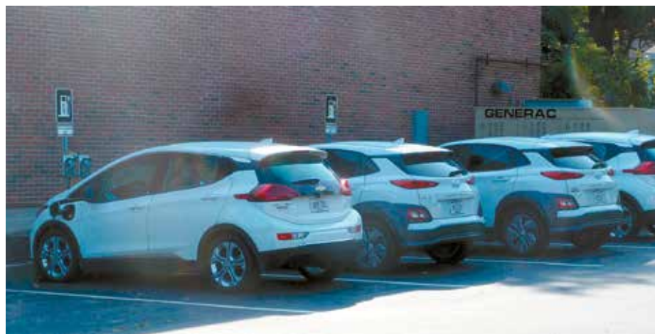
Electric Vehicles charging at Shaw Gym/Municipal Center.
