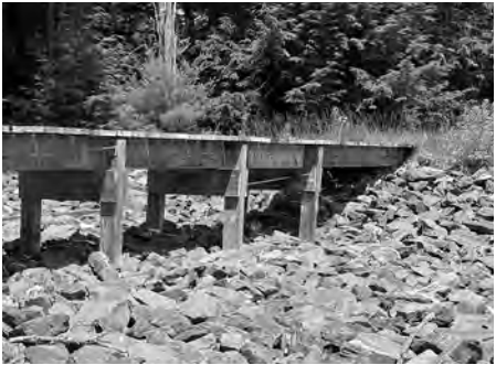
Ernie's Way showing boardwalk structure.
