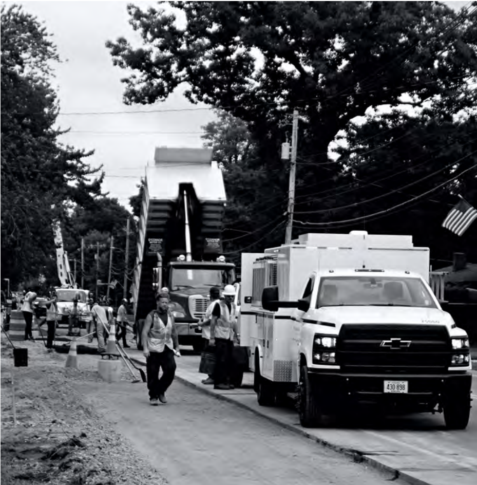
Sidewalk and electrical construction on South St. have backed up traffic coming out of or going into Gorham Center for most of the month of July. The work will continue well into August, so look for other means of getting around town if you're in a rush.
